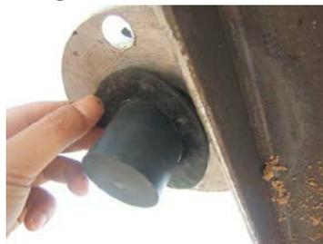
**07. Tighten nuts to fix the transducer**
